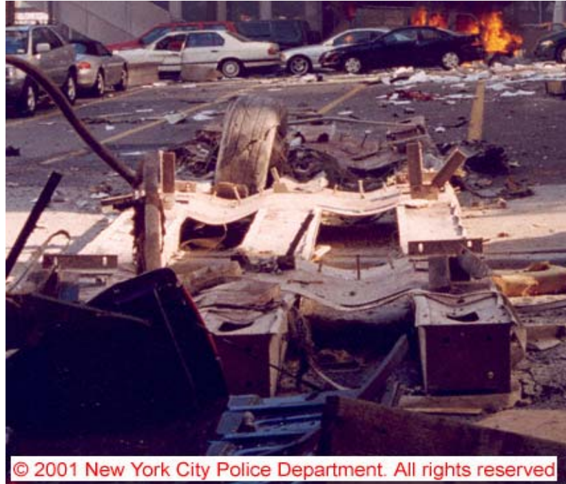
Figure 7–70. Landing gear found embedded in exterior panel knocked free from WTC 1.
