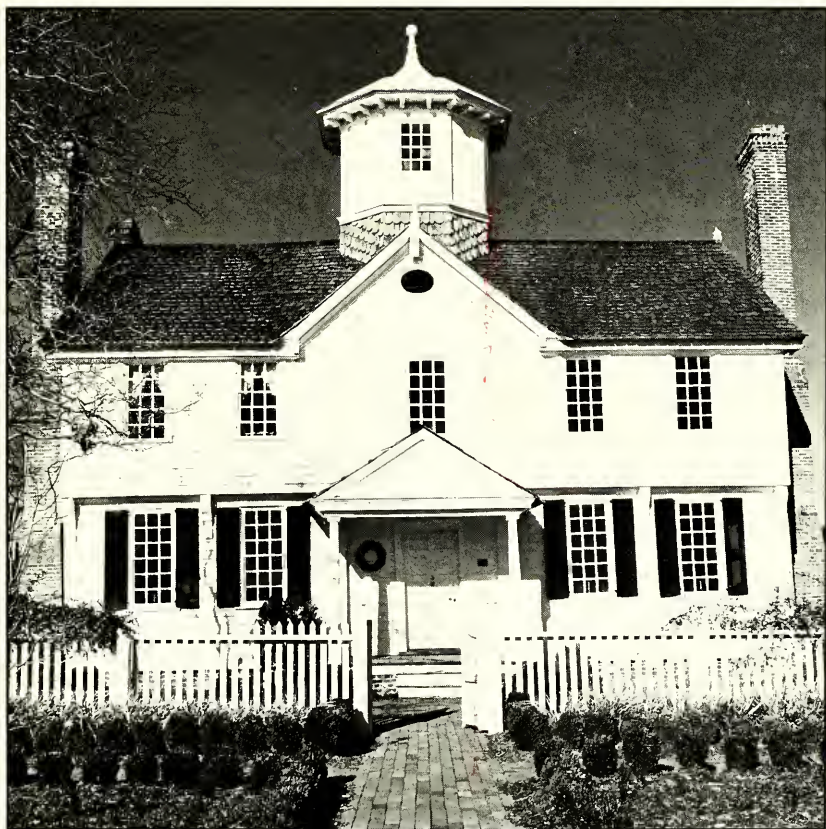
The Cupola House at Edenton, North Carolina, c. 1725 has been described as "the best example of an existing wooden house in the Jacobean tradition in all America."
