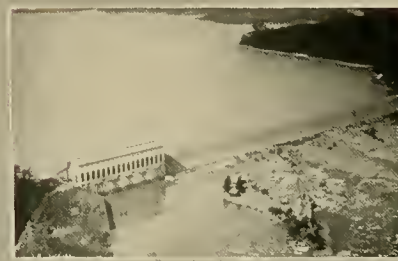
FISHING CREEK PLANT
