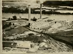
Mt. HOLLY STEAM PLANT
