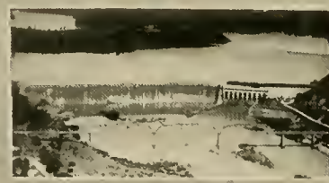
LOOKOUT SHOALS PLANT
