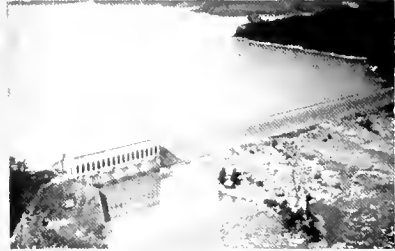
FISHING CREEK PLANT
