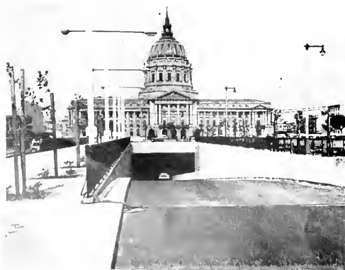
Entrance to $4,000,000 underground hall
