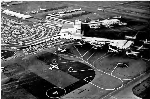
Existing terminal facilities at San Francisco International Airport showing twenty airliners at boarding positions. New concourses will soon be added to area in foreground. Partially completed pier in background will be extended to full size. Building upper left is dedicated to cargo and mail. Painted circle, center foreground, denotes helicopter landing.
