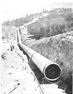
Penstock construction for Cherry Powerhouse
