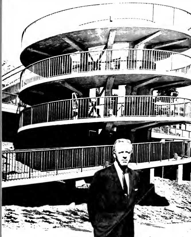
SHERMAN DUCKEL AND NEW-STYLE PEDESTRIAN OVERPASS
