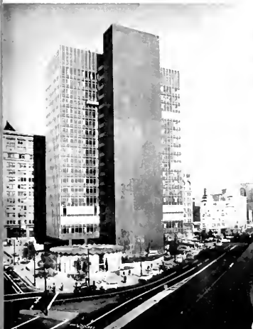
new addition to San Francisco's financial district is the 20-story Crown-Zellerbach building, with the bank-in-the-round ranch of the American Trust Company in the foreground
