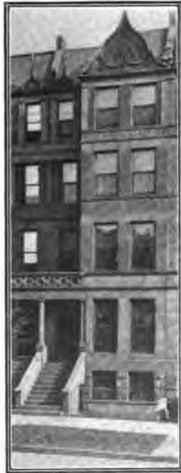
THE HUGHES HOME (West End Avenue.)
