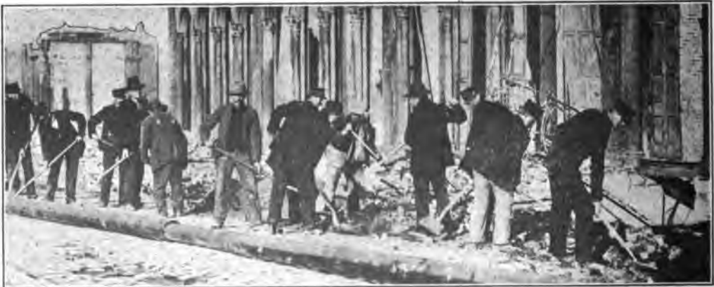
RELAYING THE FIRST CAR-TRACKS—ON MARKET STREET—AFTER THE FIRE
