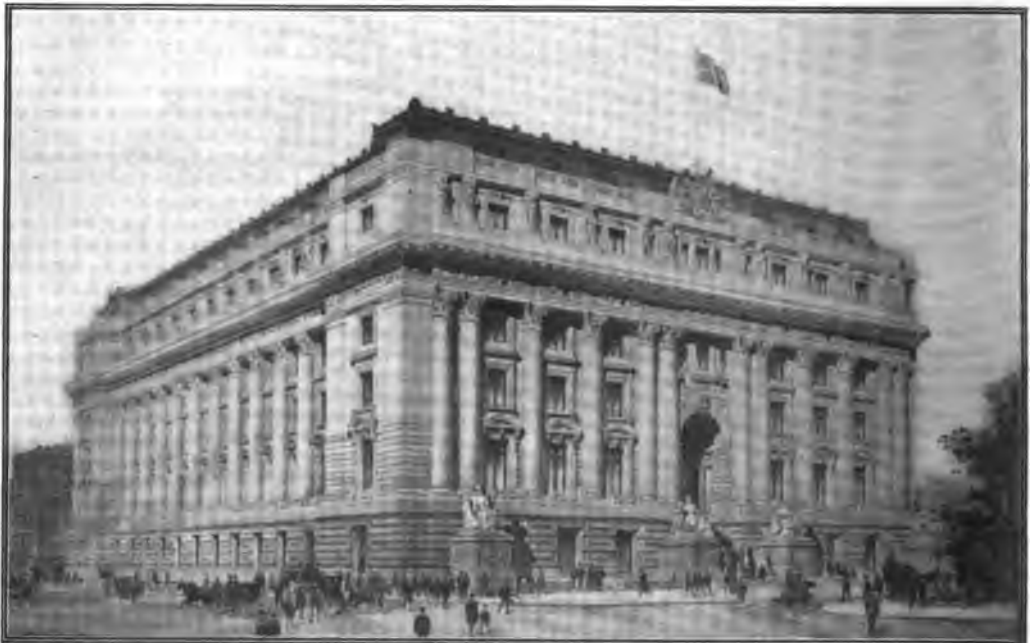
THE NEW CUSTOM-HOUSE BEING ERECTED IN NEW YORK
