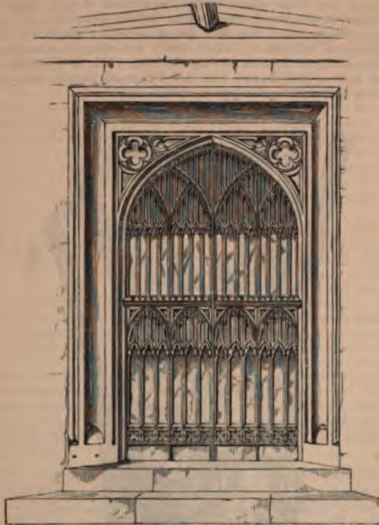
West Door, now removed, of Ewelme Church, as it was in 1834.
