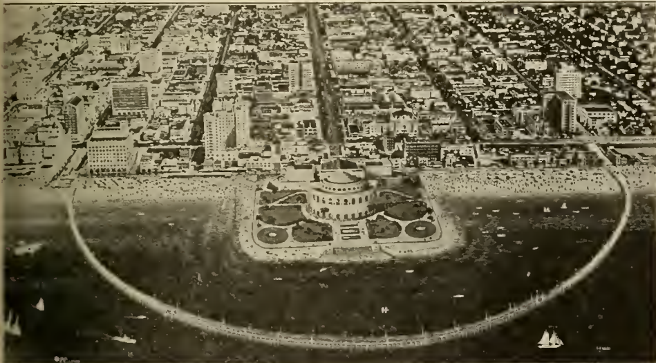
NEW $3,000,000 CIVIC AUDITORIUM AND MARINE AMPITHEATRE UNDER CONSTRUCTION.
