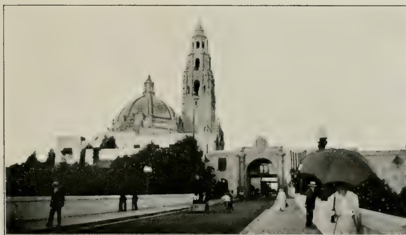
CALIFORNIA STATE BUILDING (P. C. E.)
