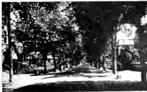
Washington Avenue and 173d Street, Before Widening
