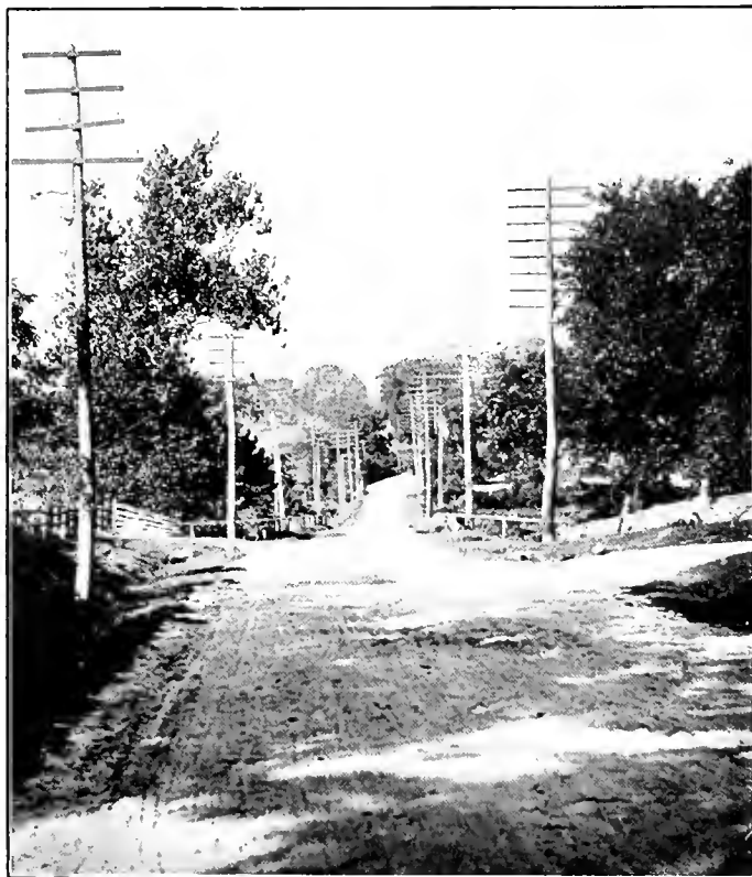
Boston Road at Spencer's Corners, near Williamsbridge
