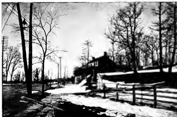
Hunt House, Boston Road
