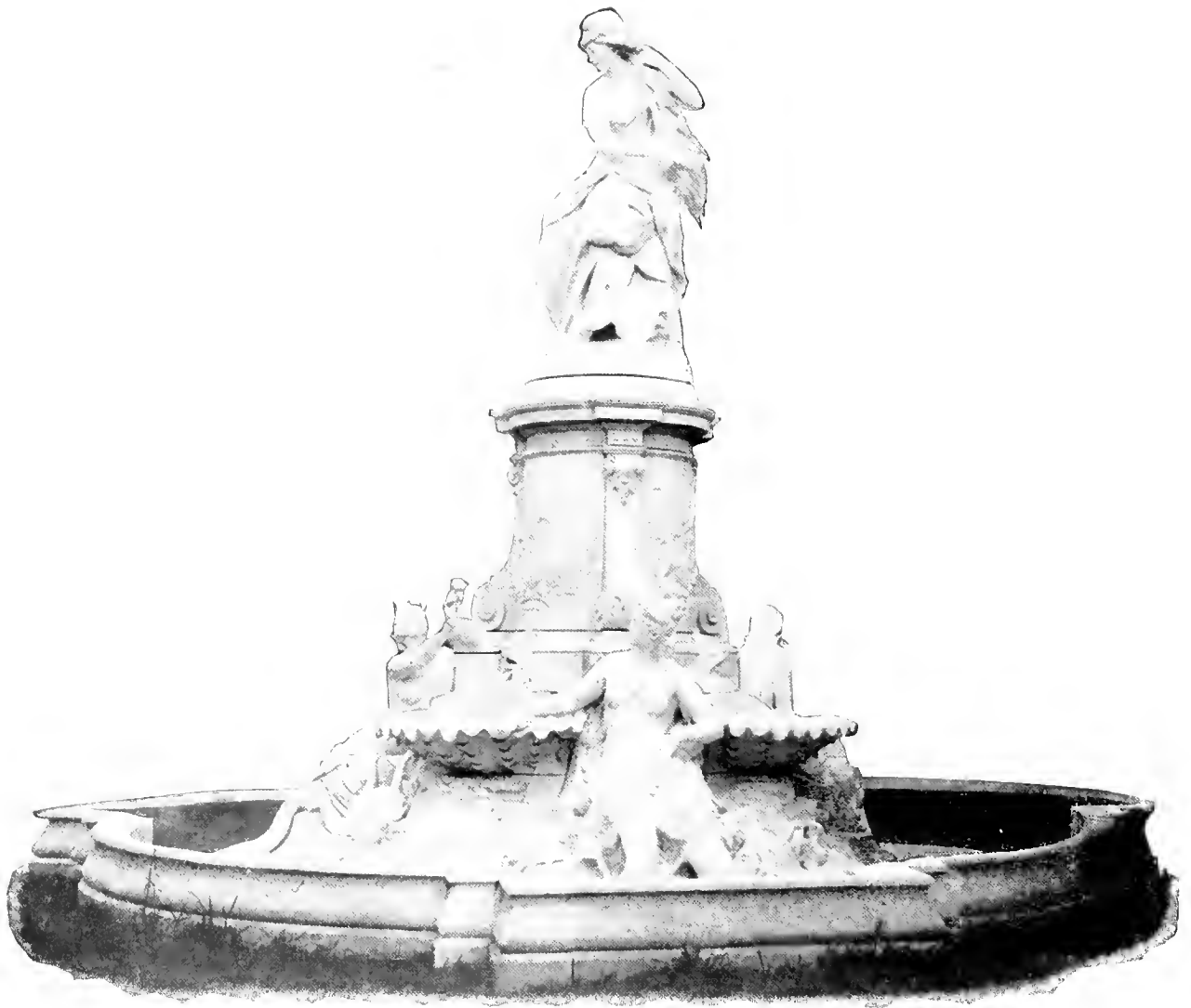
The Heine Monument, 161st Street and Mott Avenue
