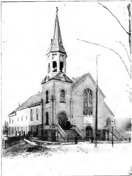
Tremont Avenue Presbyterian Church, Washington Ave., near 174th Street
