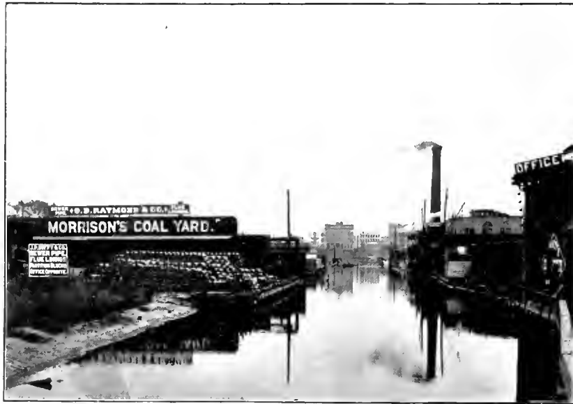
Old Mott Haven Canal, looking North from 138th Street
