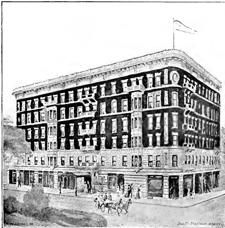
MANHASSET APARTMENT HOUSE, ERECTED BY JAMES F. MEEHAN
