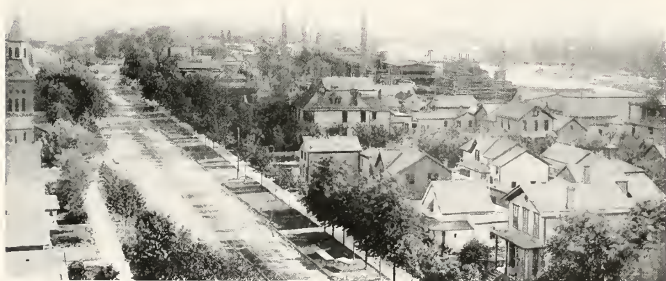
FROM THE ROOF OF THE "ACADEMY" LOOKING SOUTHWEST, 1886
