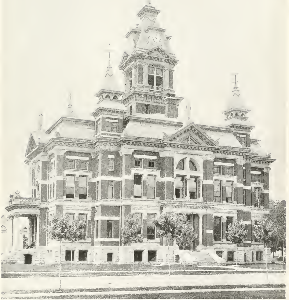
SAGINAW COUNTY COURT HOUSE, ERECTED 1884-5
