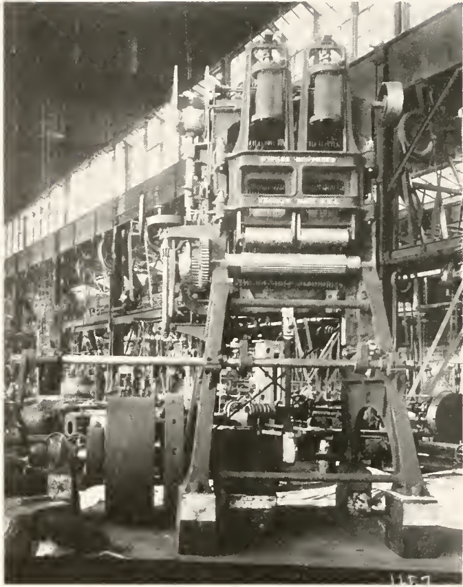
ERECTING A WICKES GANG SAW
