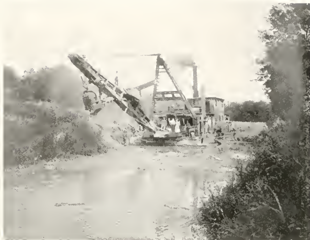
DREDGE BUILDING DIKES AT PRAIRIE FARM
