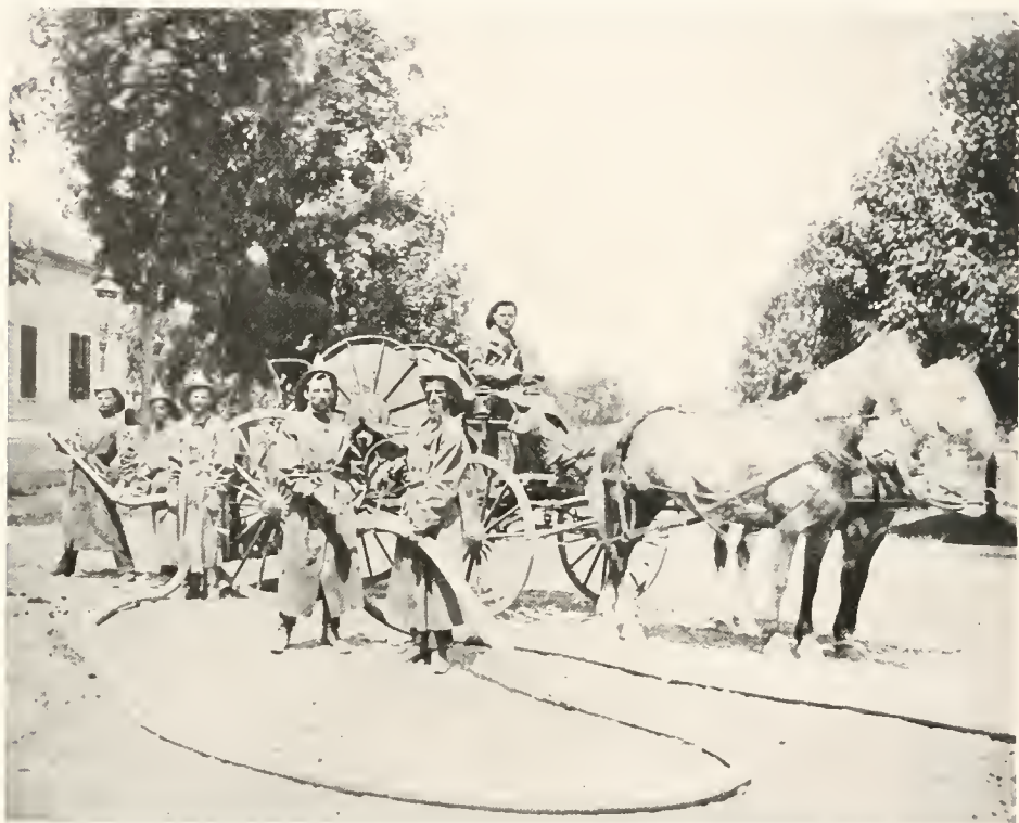
OLD STYLE HOSE REEL AND FIRE COMPANY, ABOUT 1881
