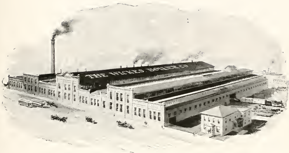
PRESENT PLANT OF WICKES BOILER COMPANY
