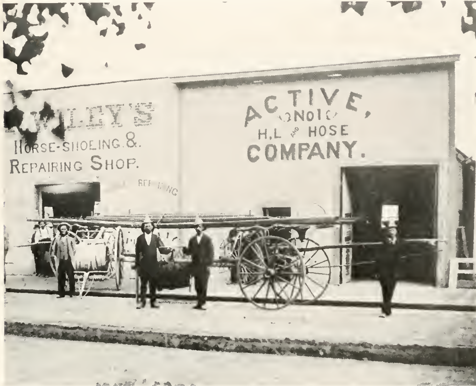
ACTIVE HOSE, HOOK AND LADDER COMPANY NO. 1
