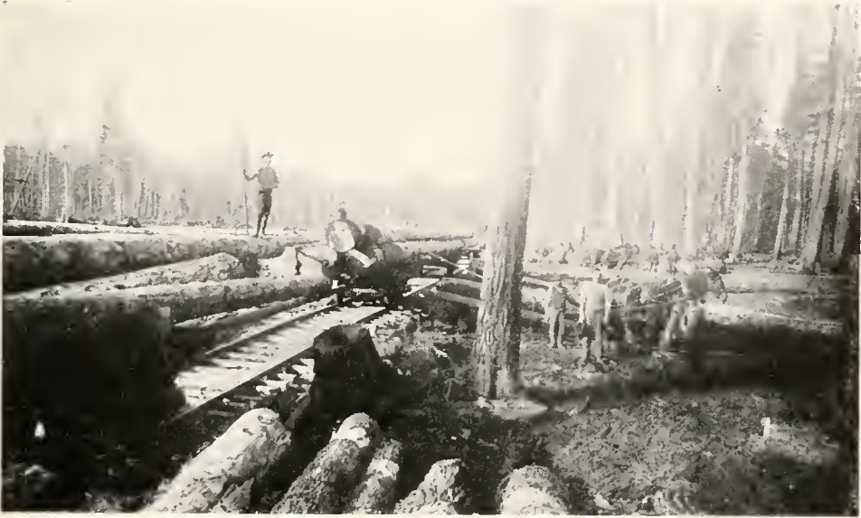
LOADING LOG TIMBER FOR SHIP SPARS
