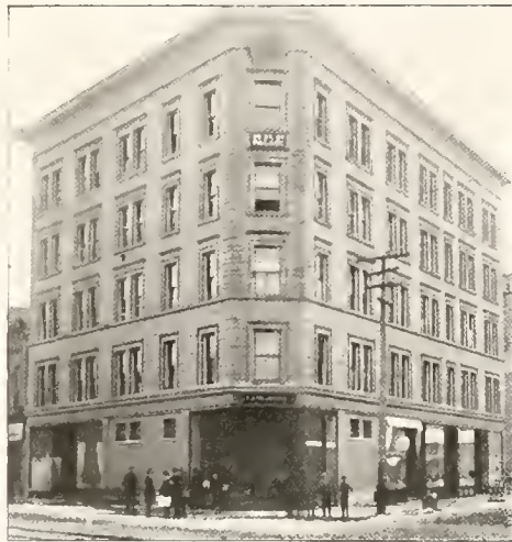
OFFICE BUILDING AT GENESSEE AND JEFFERSON AVENUES
