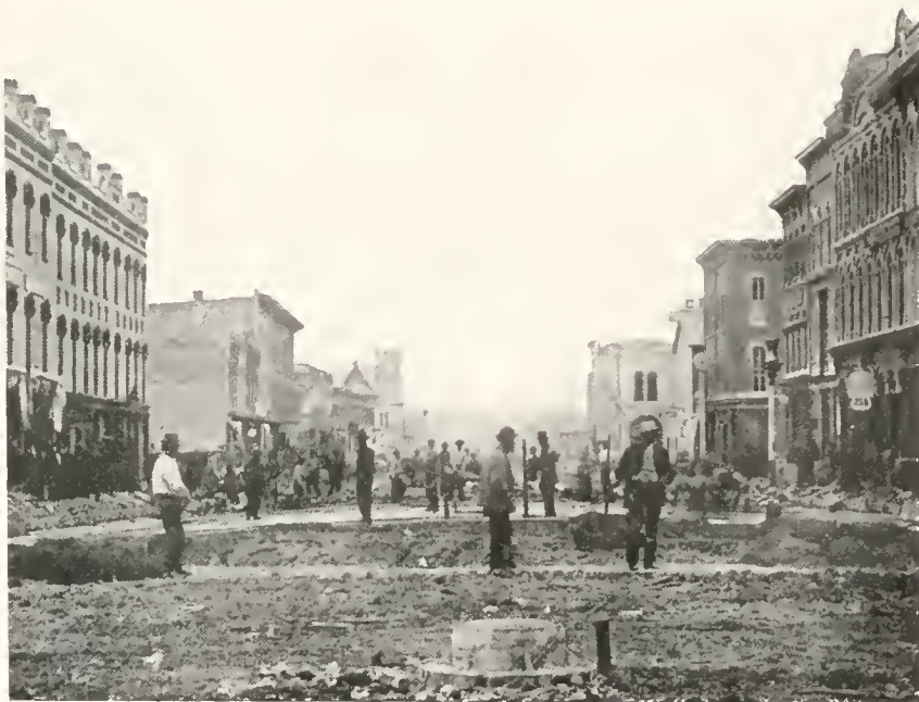
LAYING NICHOLSON PAVEMENT IN GENESEE STREET, 1868
