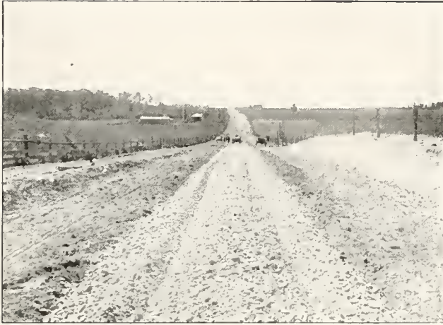
CONSTRUCTING STONE ROAD THROUGH SAND RIDGE
