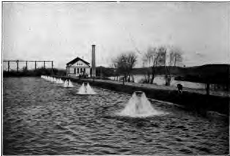
FIG. 64.—Acrators at the Albany Filtration Plant. Designed by Allen Hazen.
