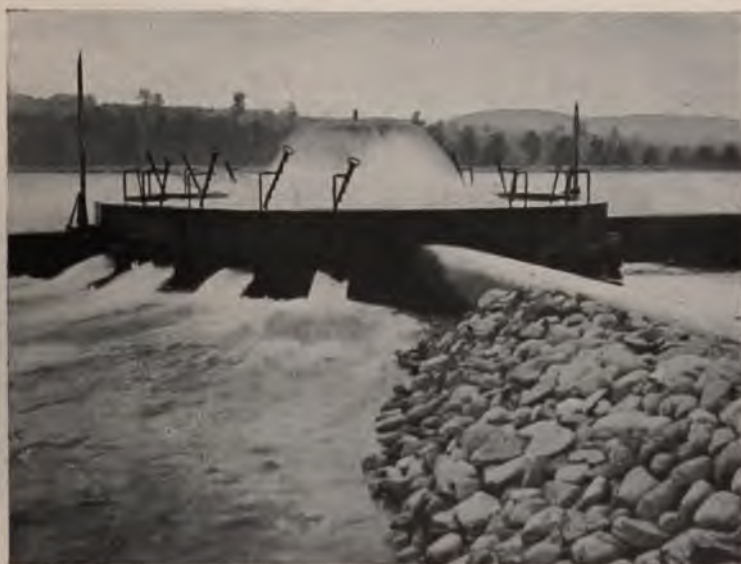
FIG. 66.—Aerator at the Ludlow Filter, Springfield, Mass.
