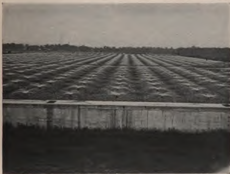
FIG. 65.—Sprinkling Filters, at Baltimore Sewage Disposal Works.
