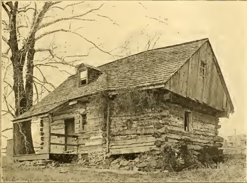
"Swedish log cabin," situated "on the west bank of Darby creek about \frac{1}{4} mile above Clifton." Photographed by C. S. Bradford and used by his kind permission. The above (built in the 18th century) shows many characteristics to be found in the log cabins built by the Swedes and Finns in their native country, the extension of the second story, "the porch-roof" etc.
