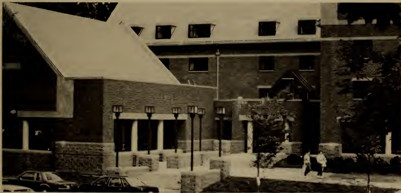
Some 225 upperclass students are the first to live in spanking-new Founders Hall, at the corner of Institute Road and Boynton Street. The complex, based on the classic architecture of WPI's first residence hall, Sanford Riley, built in 1926, features residence suites of two to three rooms; a dining room with cathedral ceiling and kitchen facilities; meeting, study and common rooms; and even a weight room in the basement. Dedication of Founders Hall was planned for Parents' Day, November 2.
